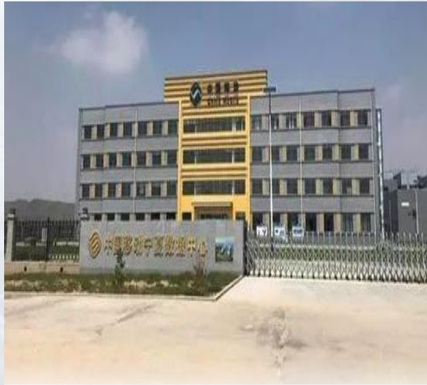
China Mobile Ningxia Data Center Project
