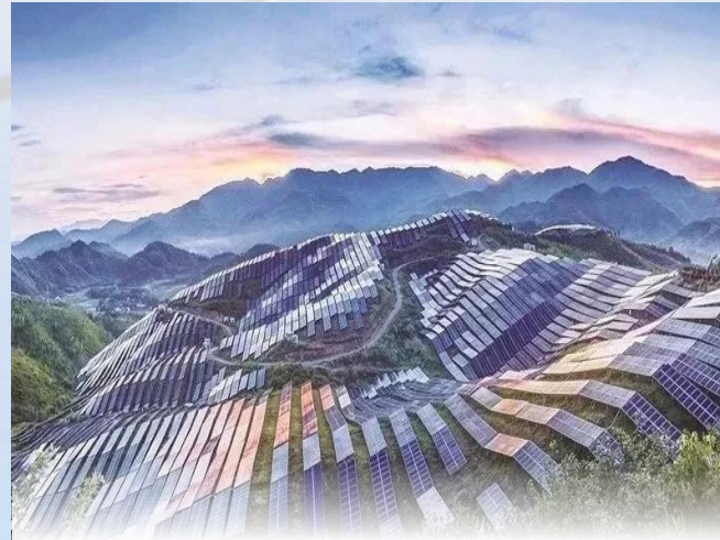
North China Power Shijiazhuang Zanhuang 250 MW Photovoltaic Composite Project
