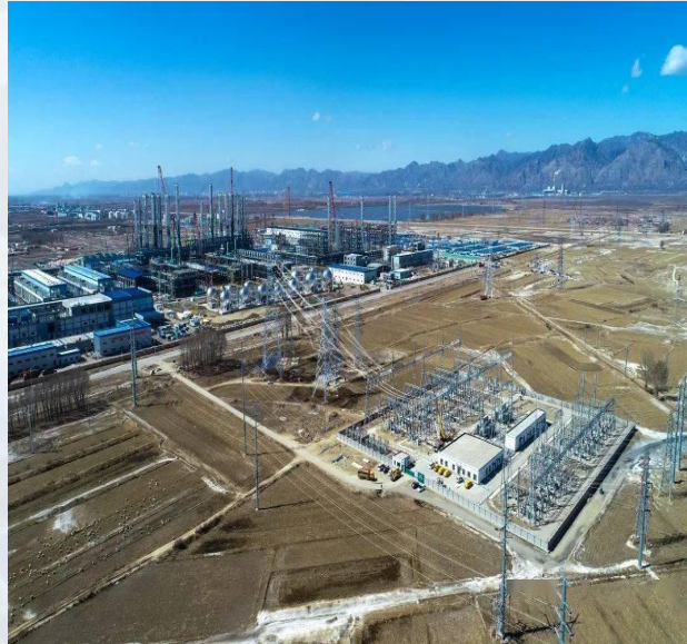
Qinghai Asia Silicon Semiconductor Company. 60000 ton electronic grade polycrystalline silicon Phase I project
