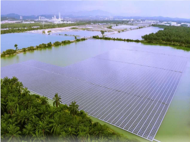
Malaysia Selangor Floating Photovoltaic Project
