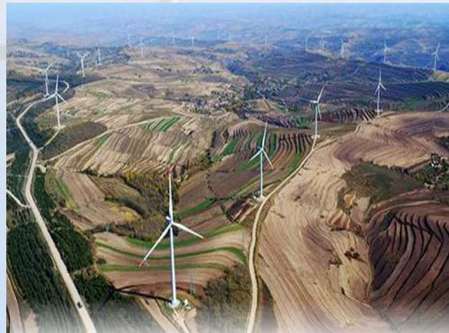
Huaneng Qidong Wind Farm Phase I
