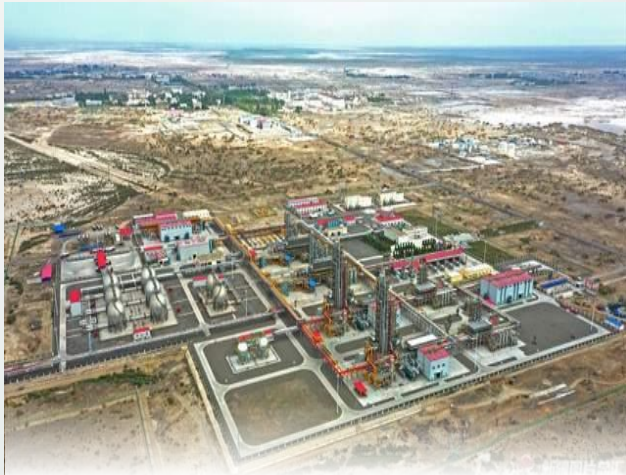
Inner Mongolia Shanghai Yicoltan Recovery Plant Project
