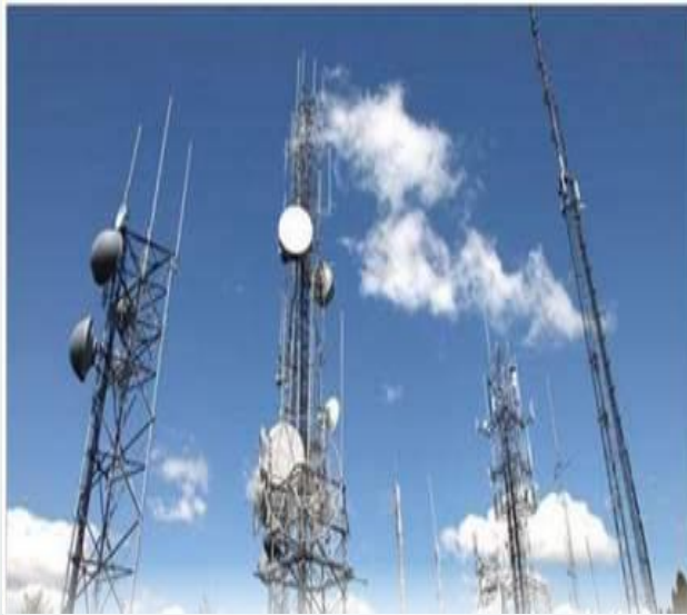
China Iron Tower Hubei Company 5G Base Station Construction Project
