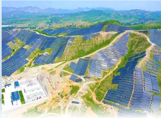
China Power Chaoyang 500 MW Photovoltaic Power Generation Demonstration Project
